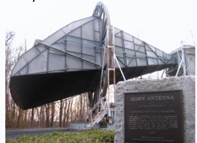
The Holmdel Horn Antenna used by Penzias & Wilson.
